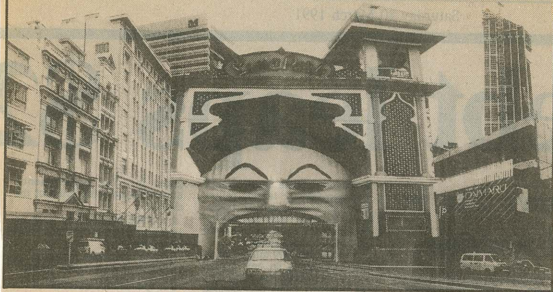
A better bridge for Lonsdale Street.
